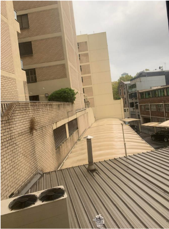
Figure 5: View north over the existing subject car park (proposed location of raised outdoor space)
