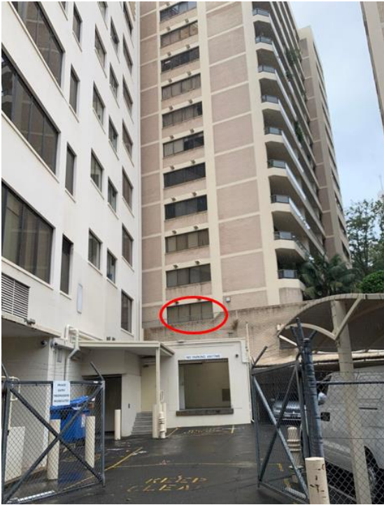
Figure 28: Existing eastern facing window of an apartment within 1 Boomerang Place.
