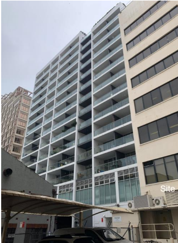
Figure 7: View southeast towards the rear of 60 - 70 William Street from the subject car park
