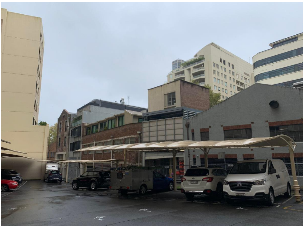
Figure 8: View east towards the mixed-use commercial buildings across Busby Lane from the subject car park
