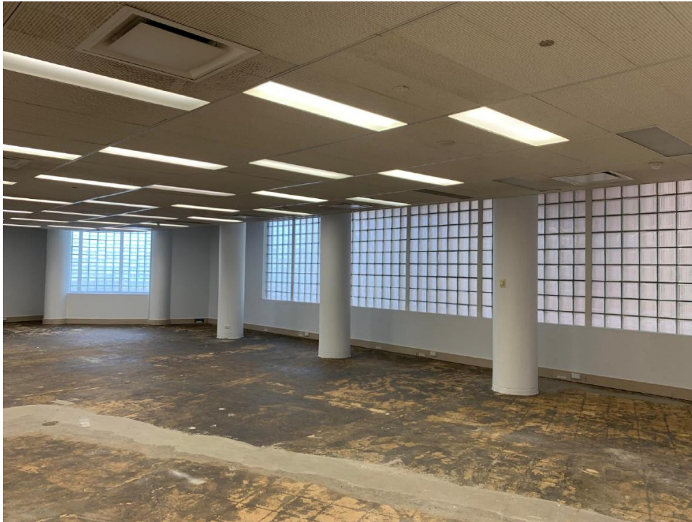
Figure 9: Internal view of subject building.
