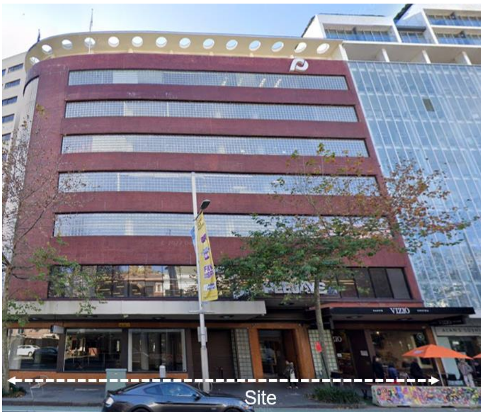
Figure 2: The site viewed from William Street
